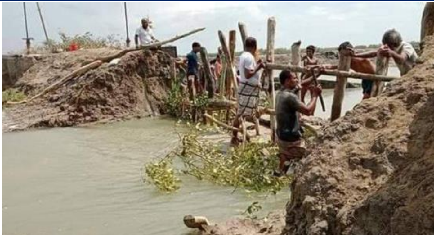
Repairing embankment following Cyclone Yaas in the south-west coast
